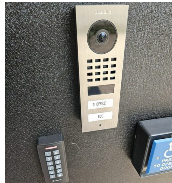
Only those authorized to be in possession of door fobs can activate the main building access control.
